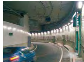
M30 Tunnel Spain
