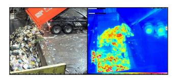
Our thermal imaging fire detection systems are a reliable choice for surveillance and recognition of spontaneous fires on conveyors, at waste transfer stations and stockpiles. The probability of spontaneous combustion in these areas is high with disastrous effects for personnel and the environment.
