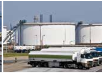
Rim Seal ... Oil Storage, Floating Roof Tanks (For SC Only)
