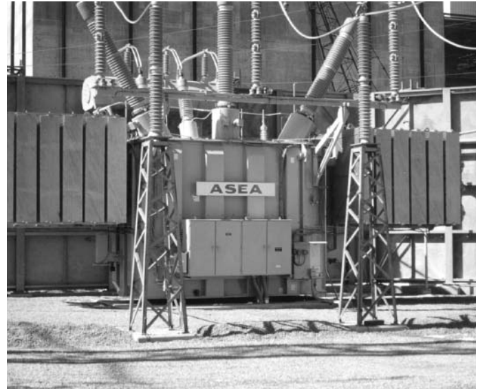
Photos taken at: Zimmer Generating Station (345/69 KV Transformer) Cincinnati Gas & Electric Co., Moscow, Ohio, U.S.A.
